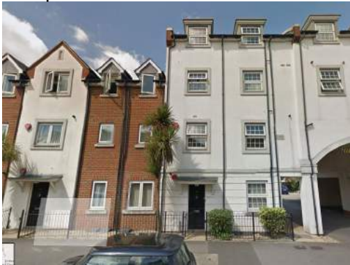
3-4 Storey Apartments - North along Silver St
