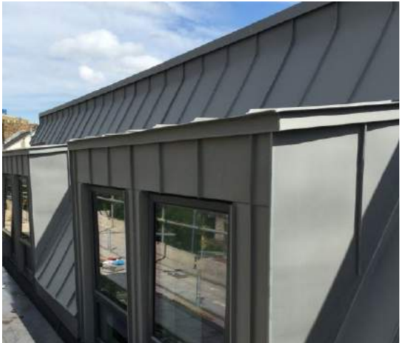
Zinc clad dormer and roof (indicative image)
