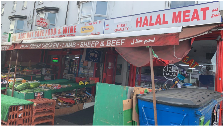
PHOTO OF EXISTING
