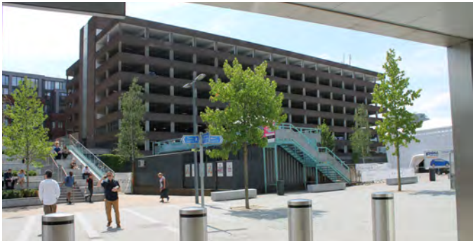
③ View from the tunnel
