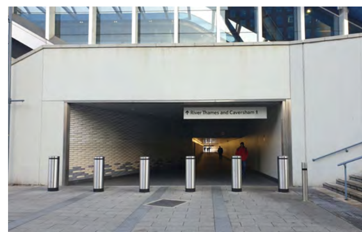
④ Tunnel entrance
