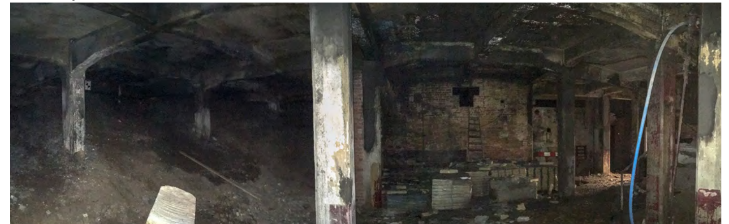
② Panoramic view of the undercroft space below Station Square
