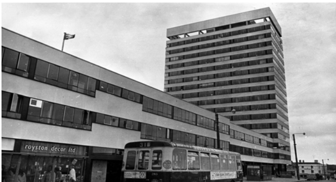
Historic image of Station Hill showing the now demolished Western Tower
