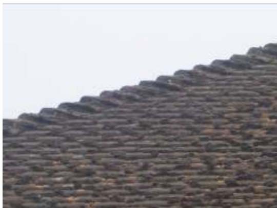
7. The hip tiles all in site and fully mortared.
