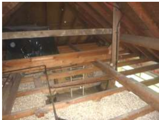
20. Section of removed ceiling in the south western corner of the loft space.
