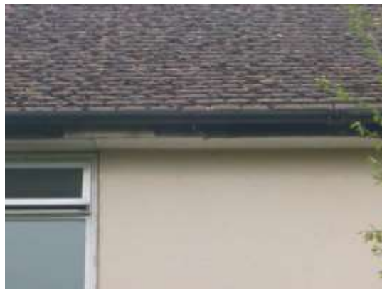
8. The complete and tightly fitted soffits.
