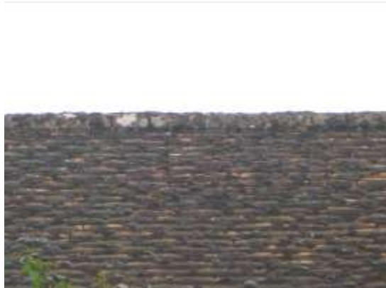
6. The flat and tightly fitted tiles and closely fitted ridge tiles.
