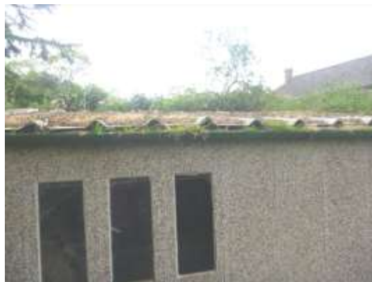
14. The garage's corrugated sheet roof.
