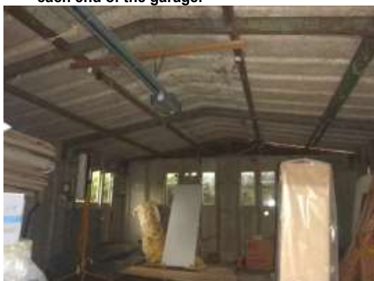
17. The interior of the garage showing the metal frame supporting the corrugated sheet roof.
