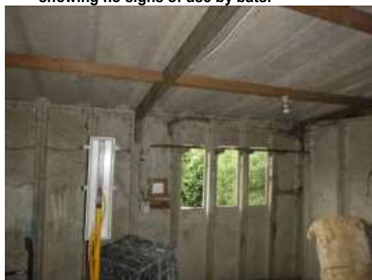
18. The pre-fabricated concrete panel walls.
