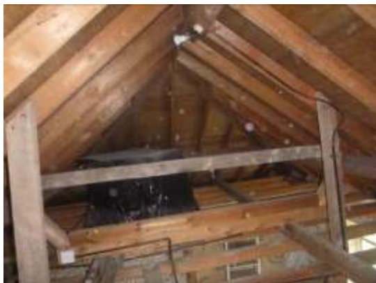
19. The loft space looking towards the southern end and the water tanks.
