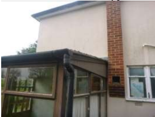
5. The single storey extension at the southern end of the house.
