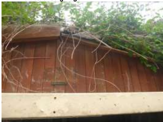
15. The tightly interlocking timber cladding at each end of the garage.
