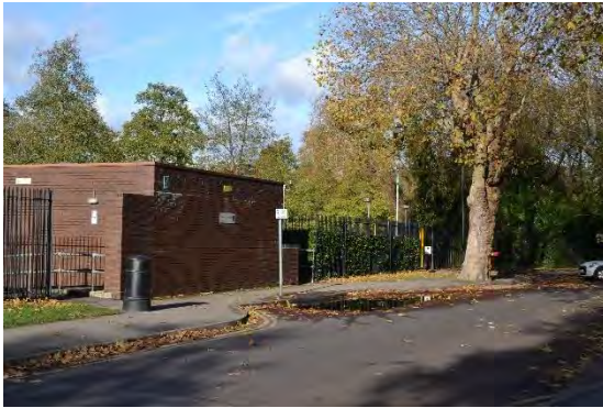
Toilet block at site entrance with site security boundary fencing adjacent
