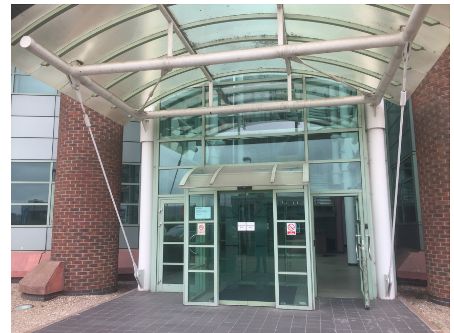
Existing view of Atlantic House entrance
