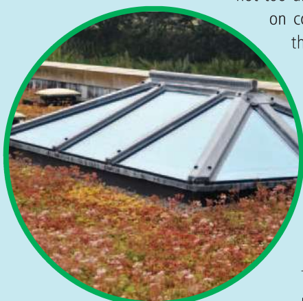
Enviromat on a flat roof.
