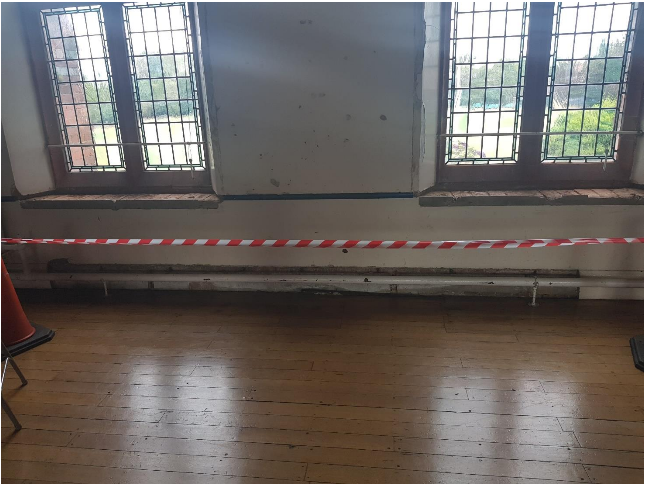
Figure 5: Showing both windows following the removal of the decayed joinery.
