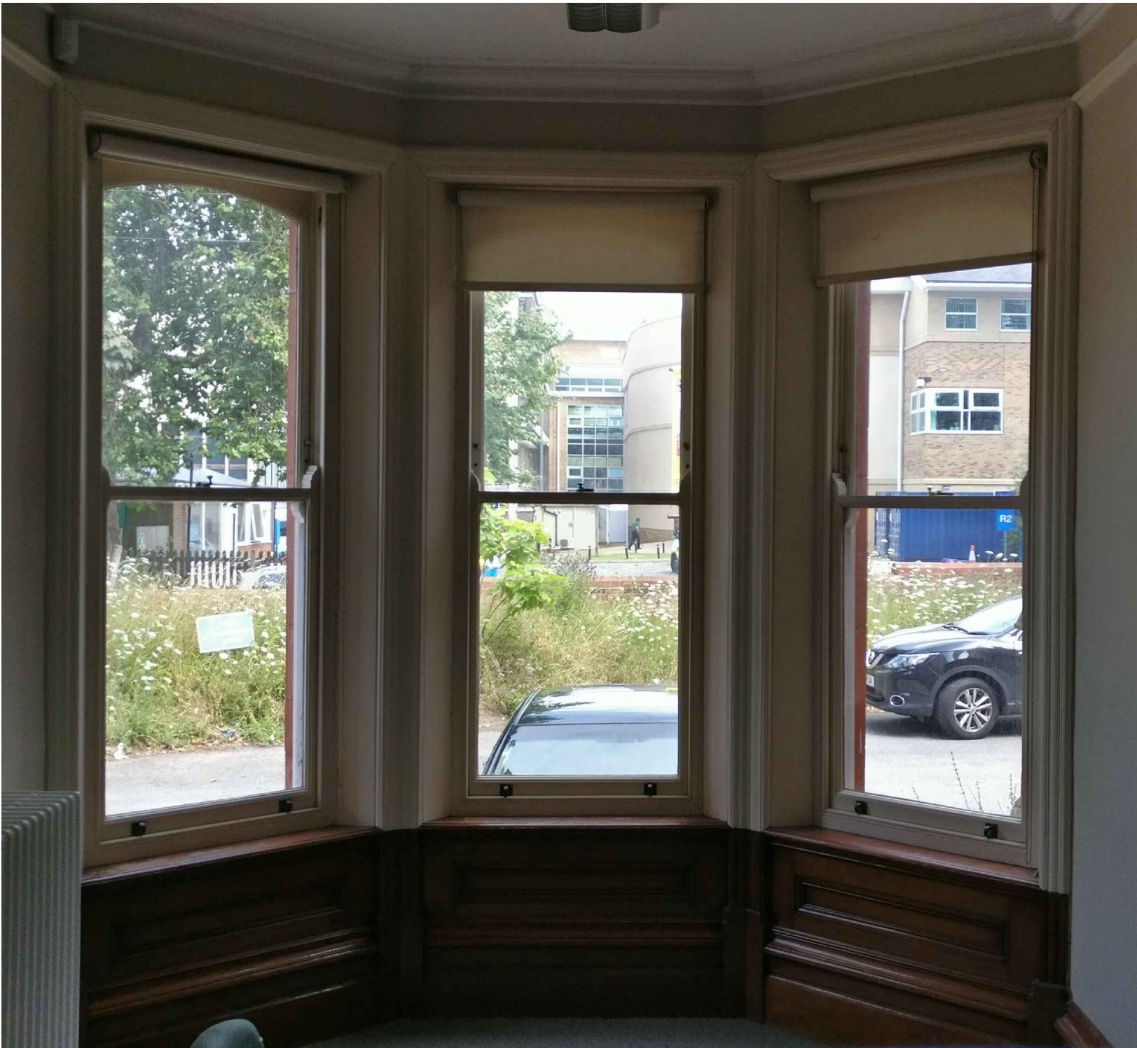
Internal Existing Photograph
