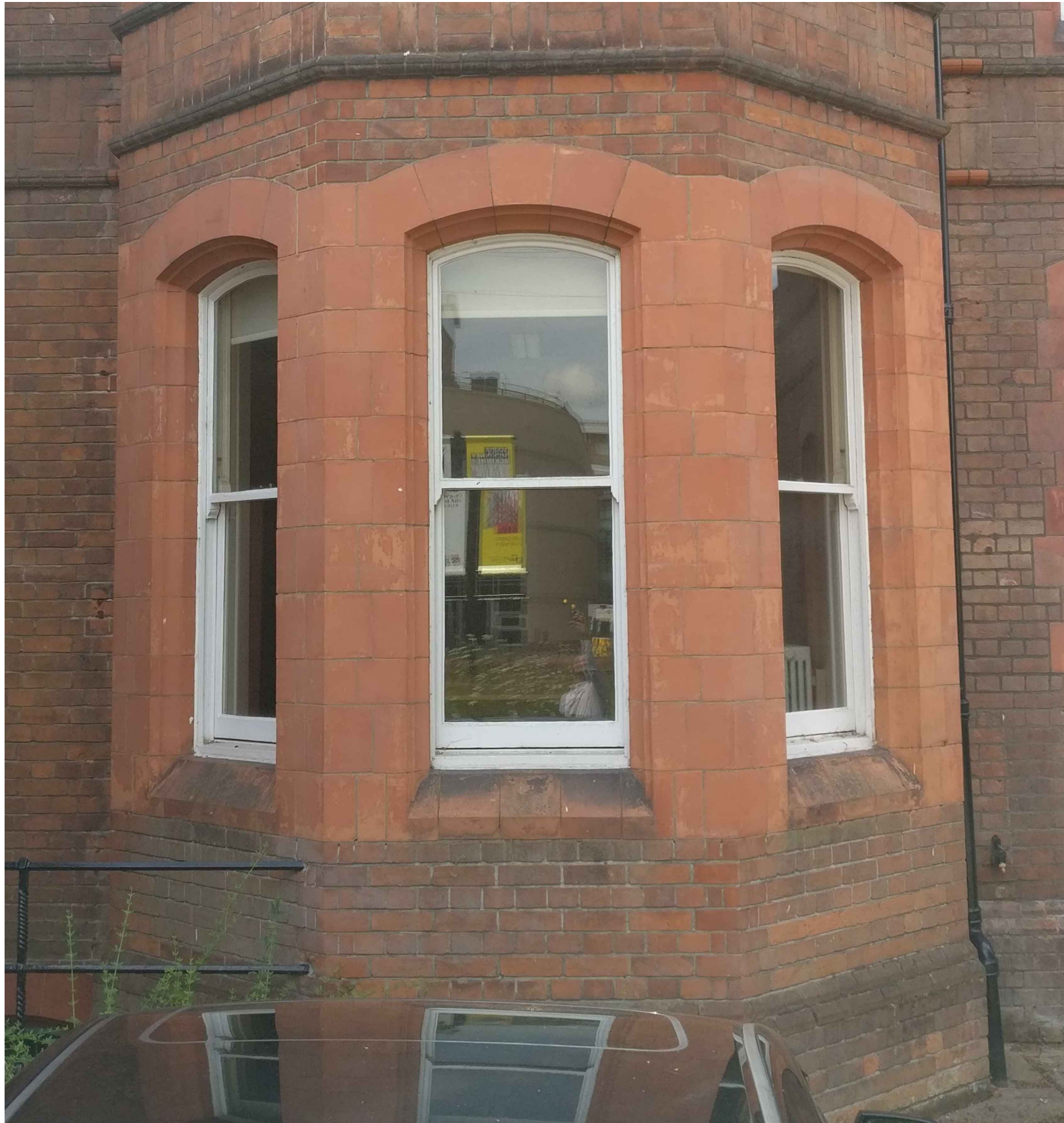
External Existing Photograph
