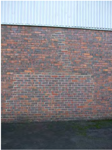
Re-pointed and patched brickwork on the exterior wall of unit 9
