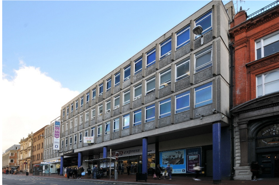
Figure 3.3: View (north) of the Market Place elevation (T P Bennett)
