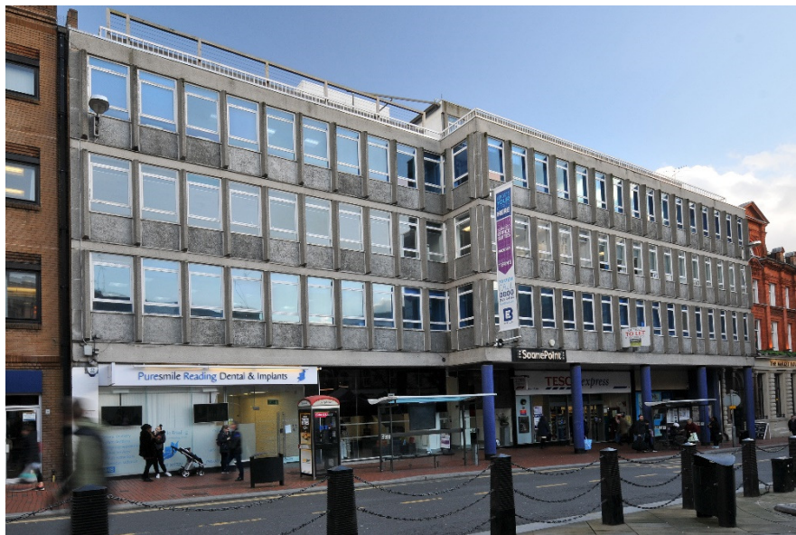
Figure 3.2: View (east) of the Market Place elevation of Soanepoint House dated 2020 (T P Bennett)
