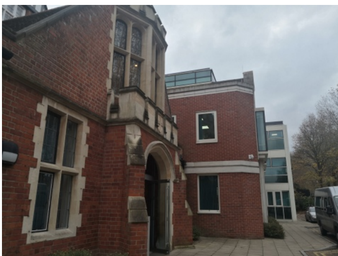
Photo 1 Front entrance of the main school building, B1, on the east of the site
