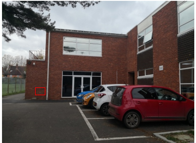
Photo 8 The south eastern corner of B1 where the classroom extension is planned. An area on the eastern facade is circled, where a hole in the brickwork is located (TN5 in the Phase 1 Habitat Plan in Appendix B)
