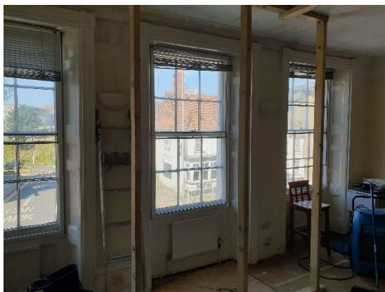
Front classroom wall plaster
