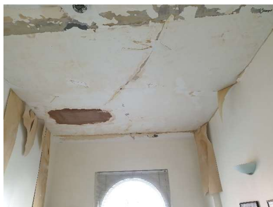
Room TR18 ceiling
