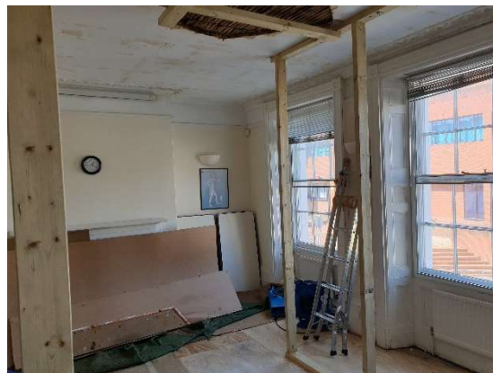
Front Classroom ceiling
