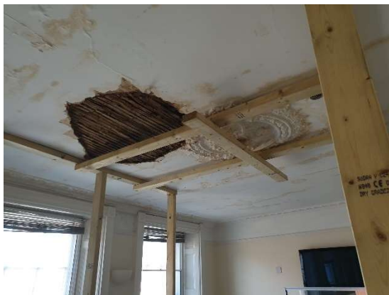
Front Classroom ceiling
