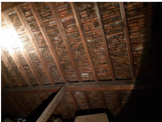
Photograph 5. The underside of the roof within the loft space of the public house (Building A).
