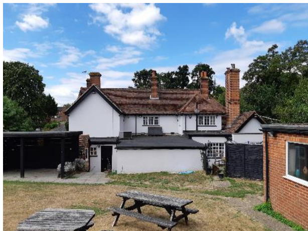
Photograph 2. The rear (north-eastern) elevation of the public house (Building A).
