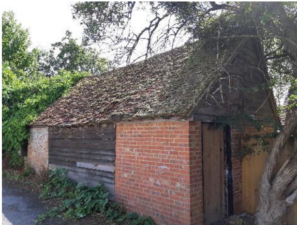
Photograph 9. The Barn (Building G) viewed from the west.
