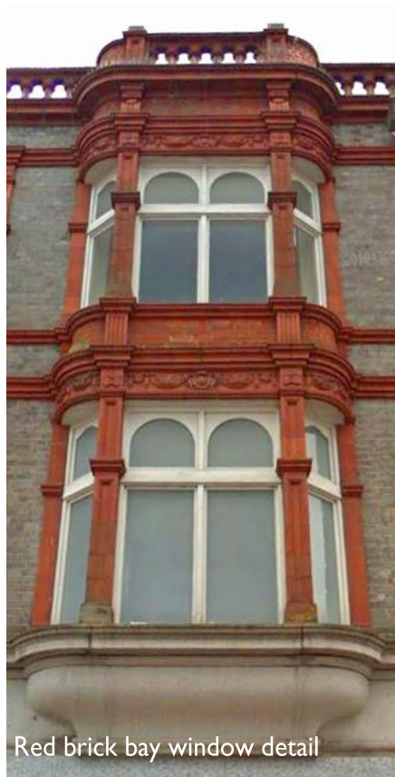
2. 173 Friar Street: Façade Detail
