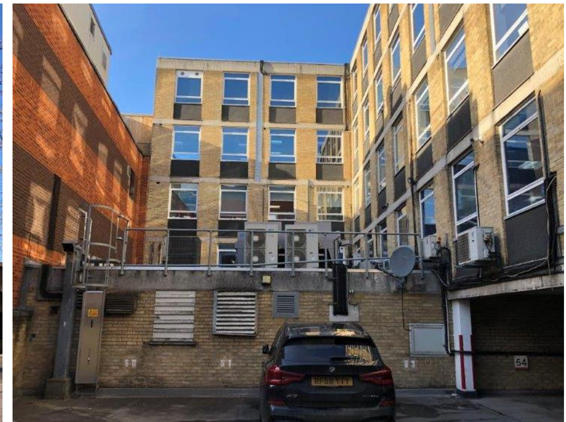
Internal courtyard Façade on Ground Floor Car Park Level
