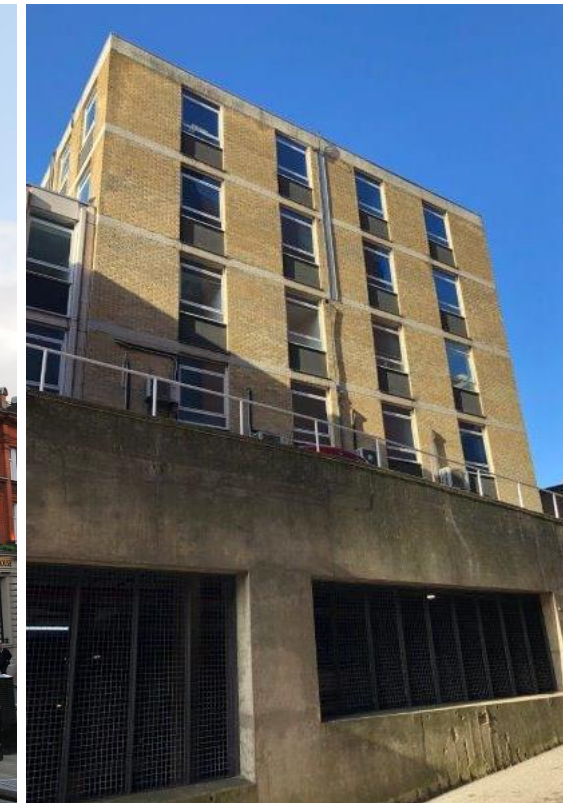
Rear Façade facing the Regus Building
