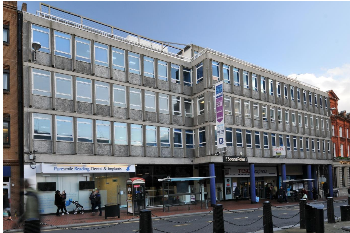
West Facing Façade onto Market Place Square
