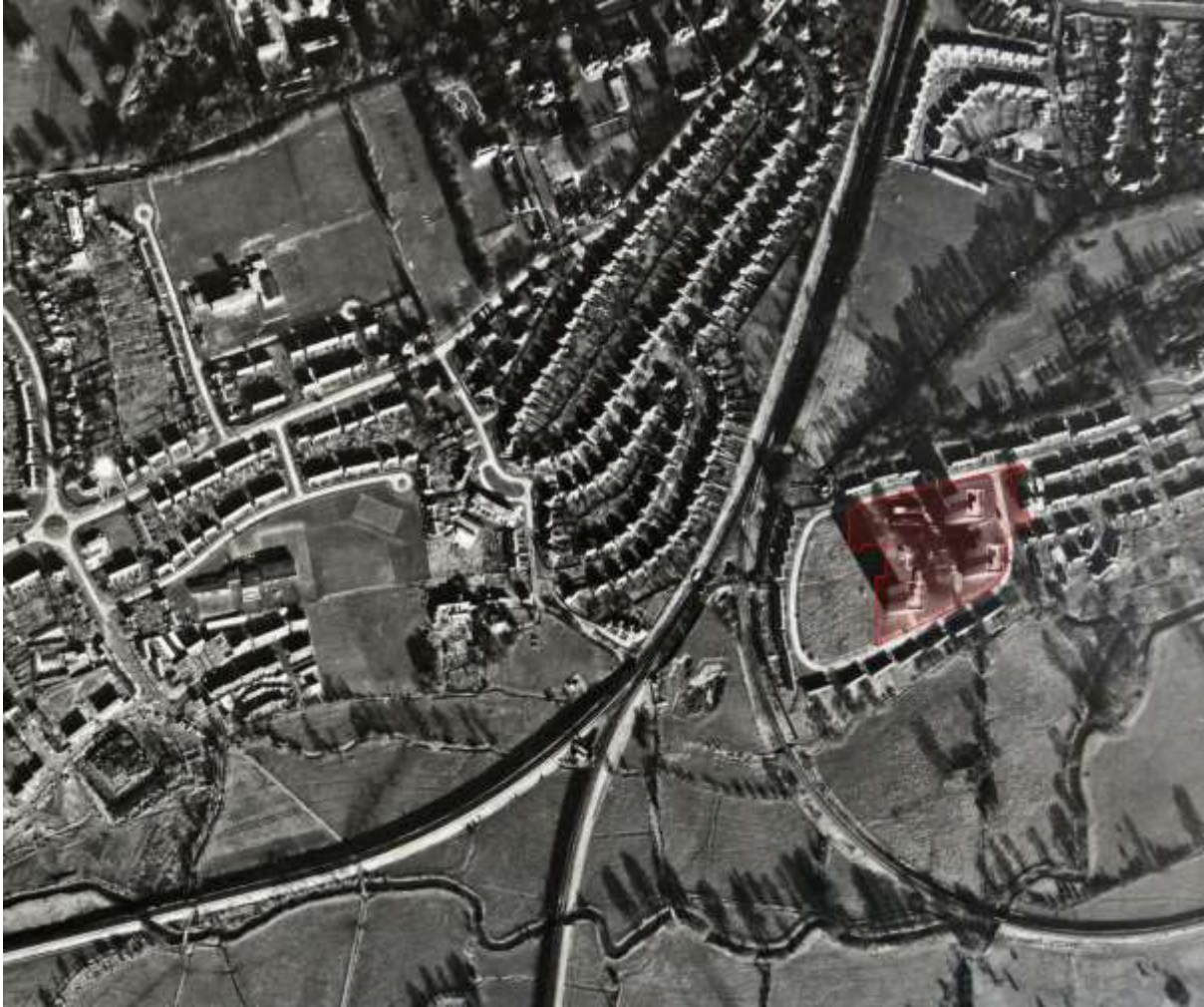
Figure 17: Aerial photograph taken in 1964, with the site outline in red
