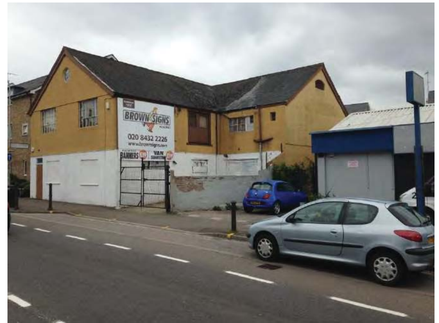
Derelict industrial unit to the south east of the site
