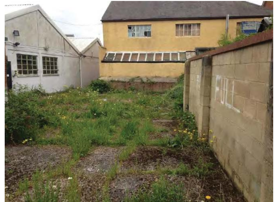
Southern part of the site – on-site chimney and area of former structure
