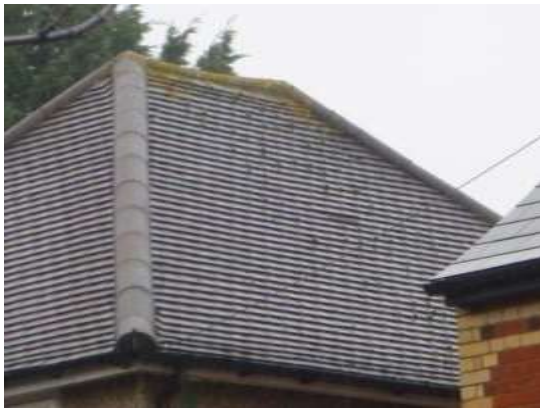
3. The tightly fitted roof tiles.
