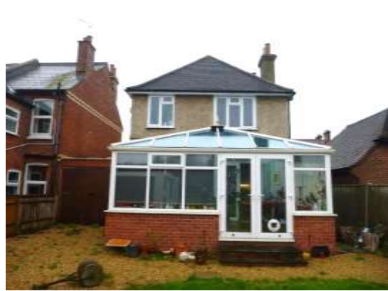
2. Rear of the building viewed from the north.
