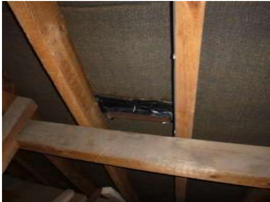
11. The gaps cut into the felt for the vents.
