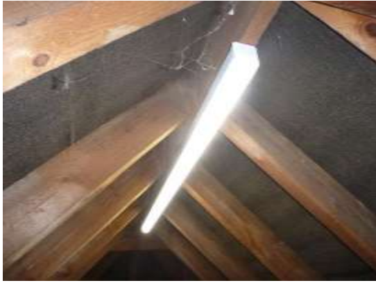
13. The cobwebbed ridge beam.
