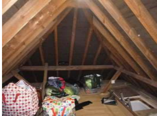
10. The roof space.
