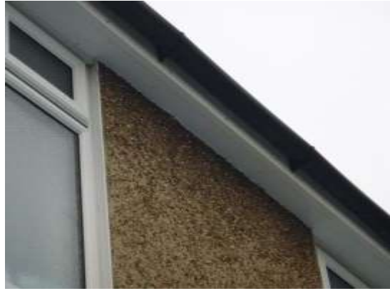
8. The tight soffit boxes at the eaves of the house.
