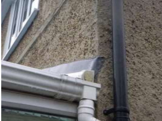
9. The tight lead flashing at the junction between the conservatory and the external wall of the house.
