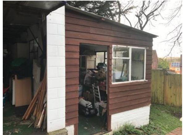
Photograph 2: South east aspect of the utility room with wooden cladding
