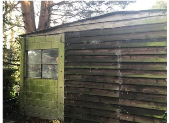
Photograph 4: North west aspect of the building
