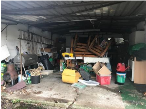
Photograph 3: Internal view of the garage
