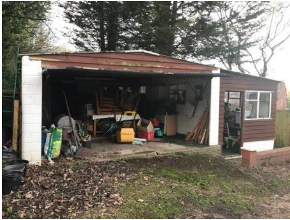
Photograph 1: South east aspect of the building showing garage and utility room
