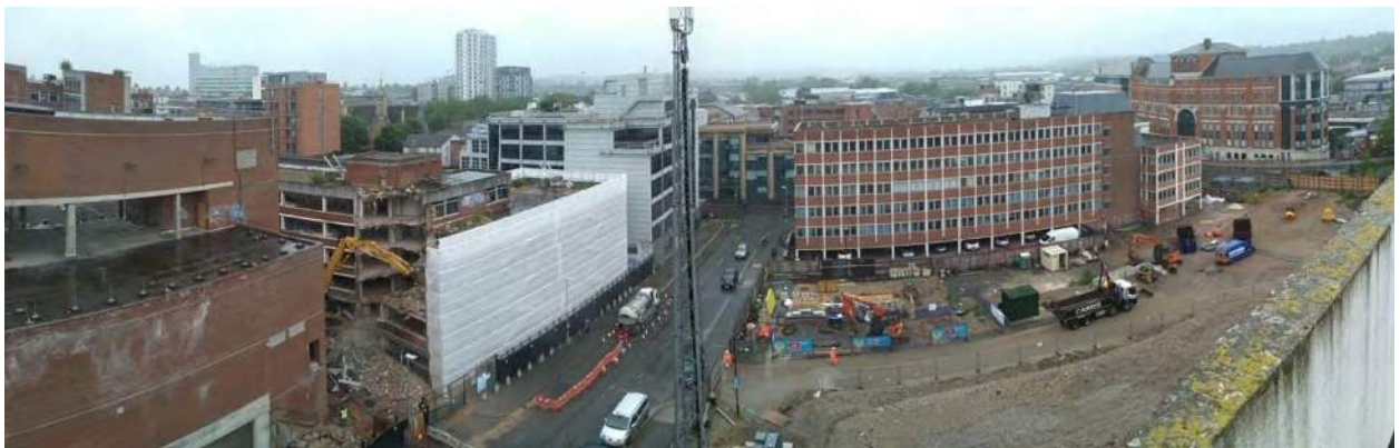
Plate 12: NCP car park upper level looking north-east
