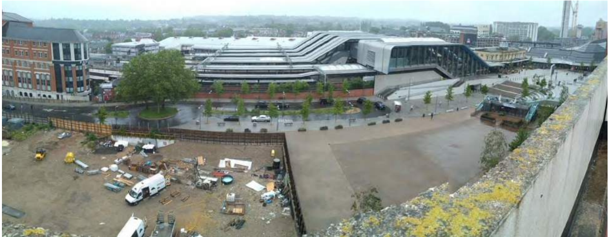
Plate 11: NCP car park upper level looking north-east
