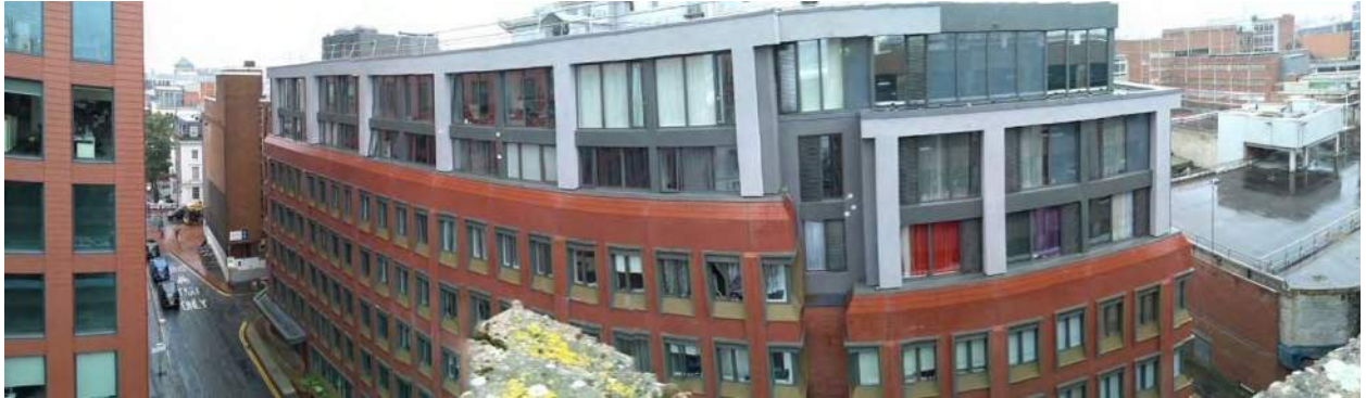
Plate 13: NCP car park upper level looking south
