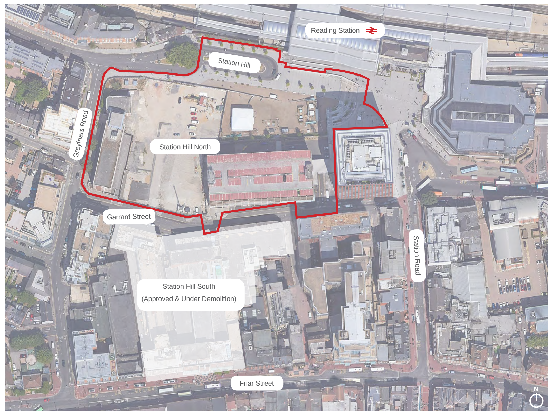
Station Aerial View: The red line indicates the approximate extent of this hybrid planning application for the North Site
