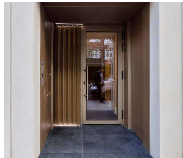
Recessed communal entrance
