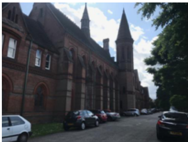
Photo 4 – Northern elevation of the Waterhouse Building
