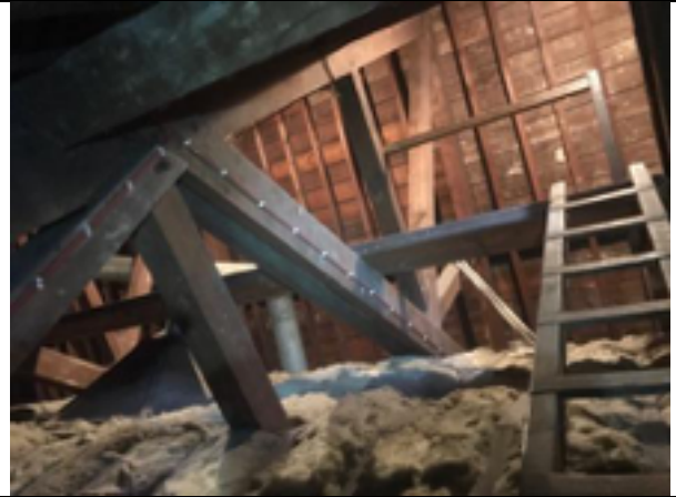
Photo 17 – Internal photo of central loft void (Loft 4)
