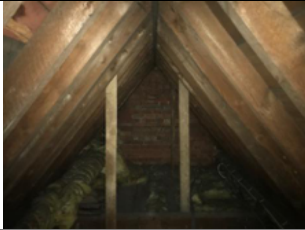
Photo 16 - Internal photo of loft void
