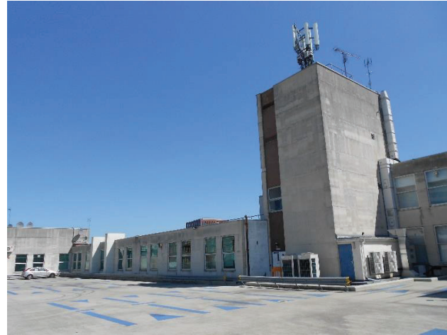
Photograph 7 View of western elevation of Quadrant House on top of Broad Street Mall.
