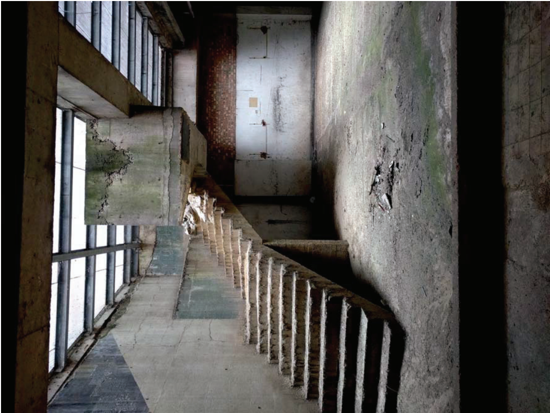
Fig 12 North west facing view of basement at road Street Mall (MO A photograph, 2 /06/201 )
