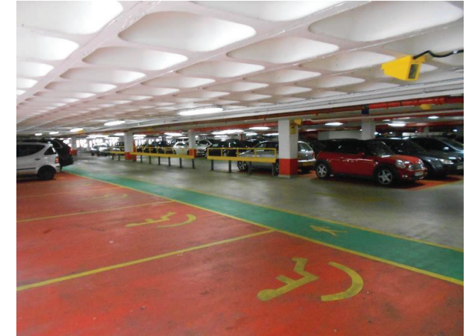
Photograph 10 View of interior car parking areas
