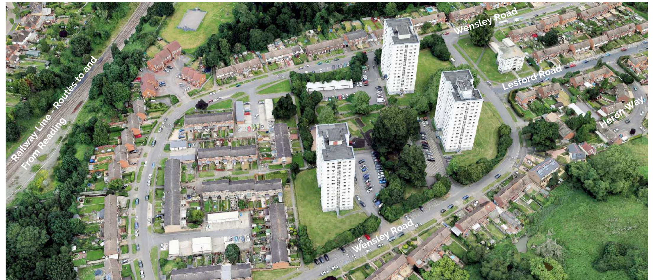
Existing Aerial Photo from the South
