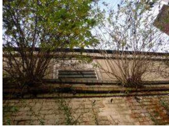
2. The southern side of the building.
