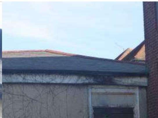
8. The flat slate roof tiles and mortared hip and ridge tiles.
