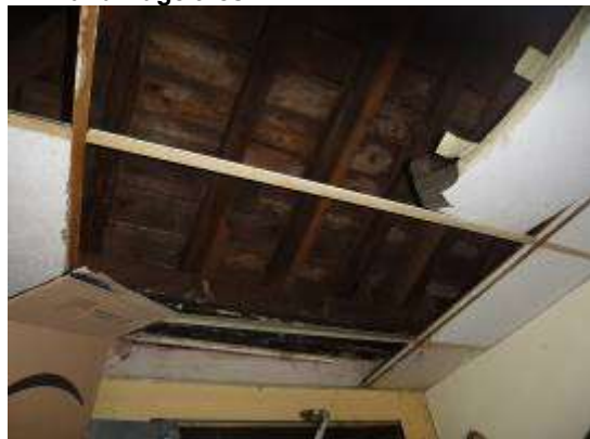
10. The view of the underside of the roof space in the north eastern corner of the building.
