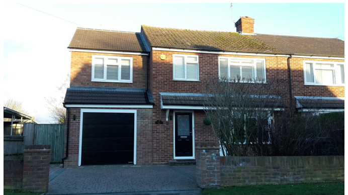
88 Woodcote Way – existing two storey side extension
