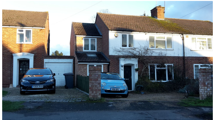
68 Woodcote Way – existing two storey side extension
