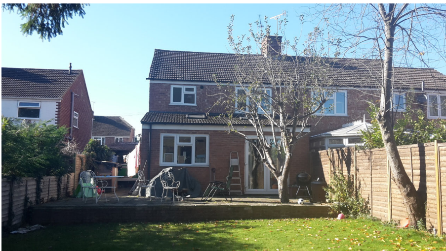
66 Woodcote Way – Rear elevation illustrating existing single storey rear extension
