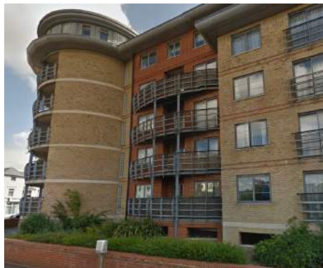
5-6 Storey Apartments at Silver St
