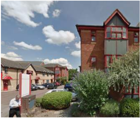
3 Storey Windsor Court - Opposite the site
