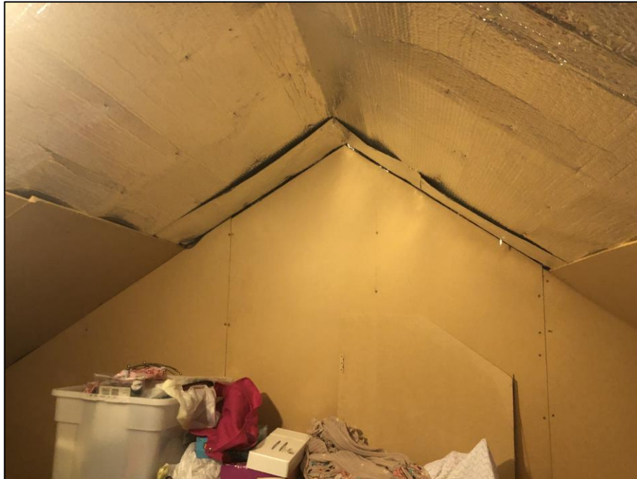
Plate 3 – Internal view of loft space
