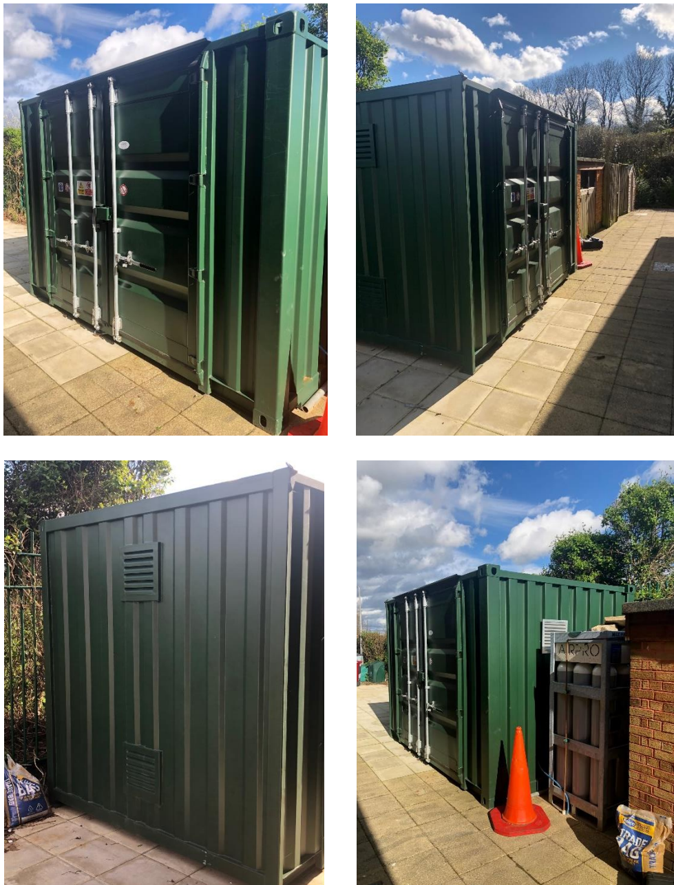
Figure 5.1 Photos of enclosure
