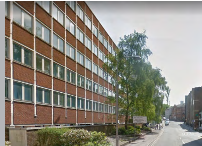
Existing condition Greyfriars Road
