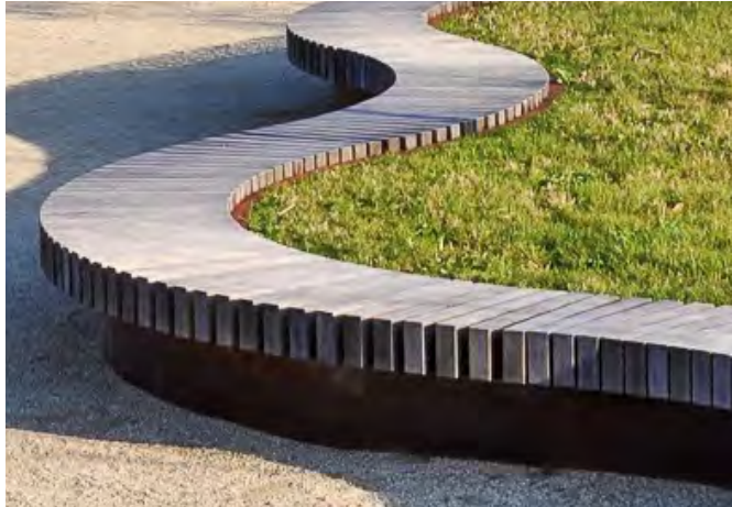
Timber Tops to Benches
