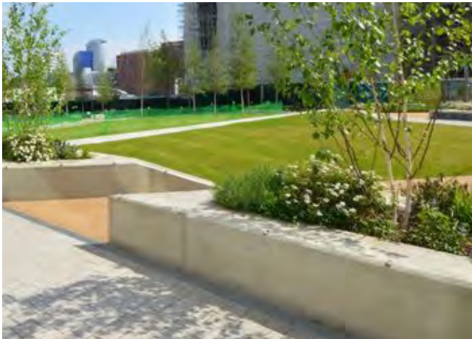
Retaining Concrete Edge ■
