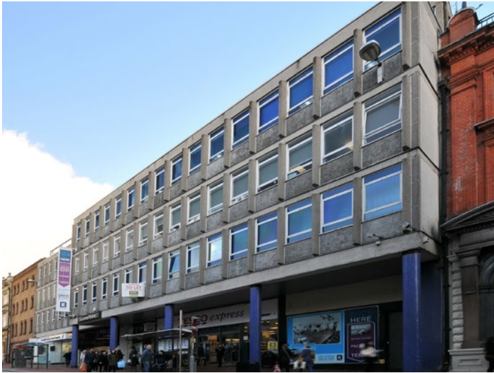
4. The building occupying the Site and its frontage with Market Place
