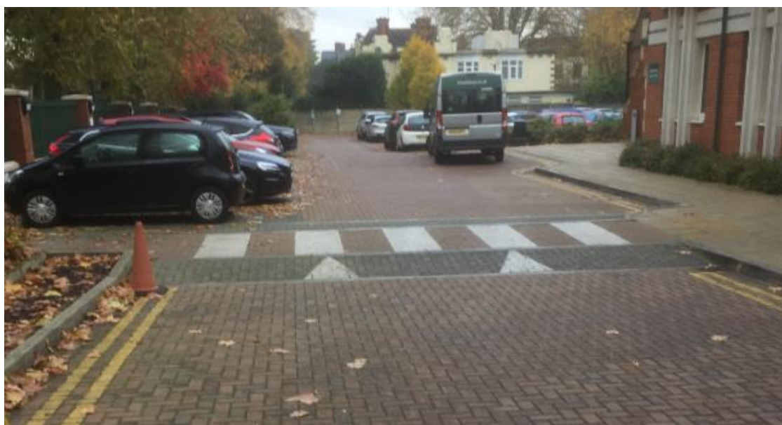
Figure 3.6 – Raised Crossing within Senior School Car Park.
