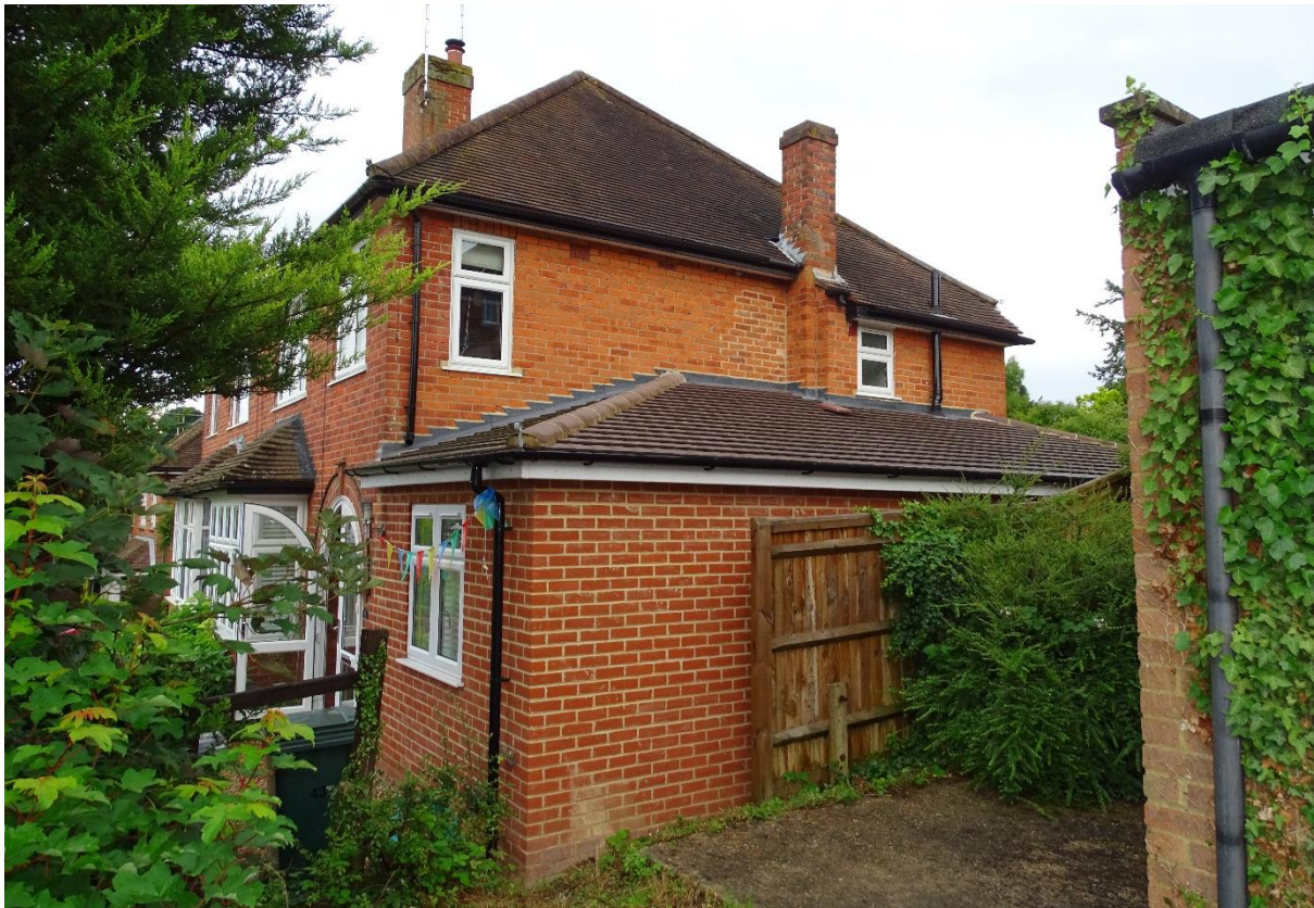
Image 2 – West facing elevation of the property
