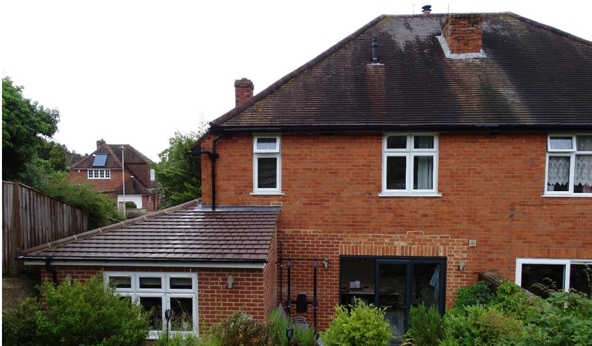
Image 4 – Rear South facing elevation of the property
