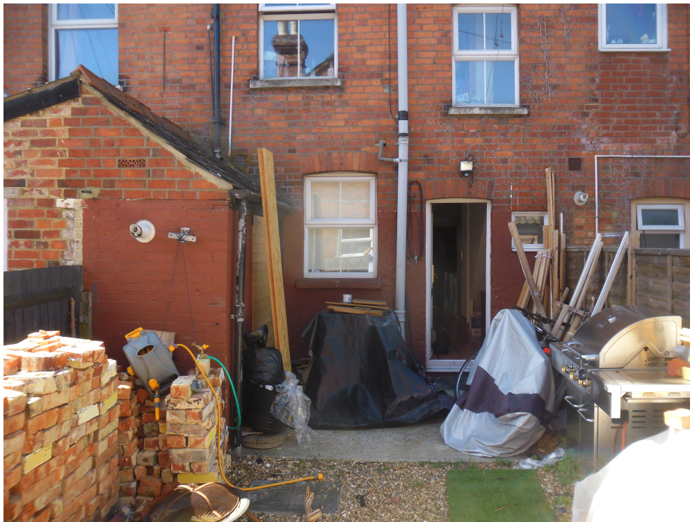
Photograph of existing rear façade (1)
