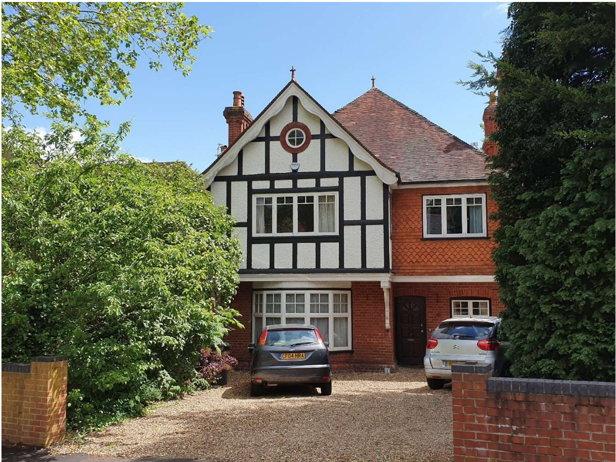
PHOTO No.878-08: 26 Kidmore Road opposite the site. Large roof, high ridge.
