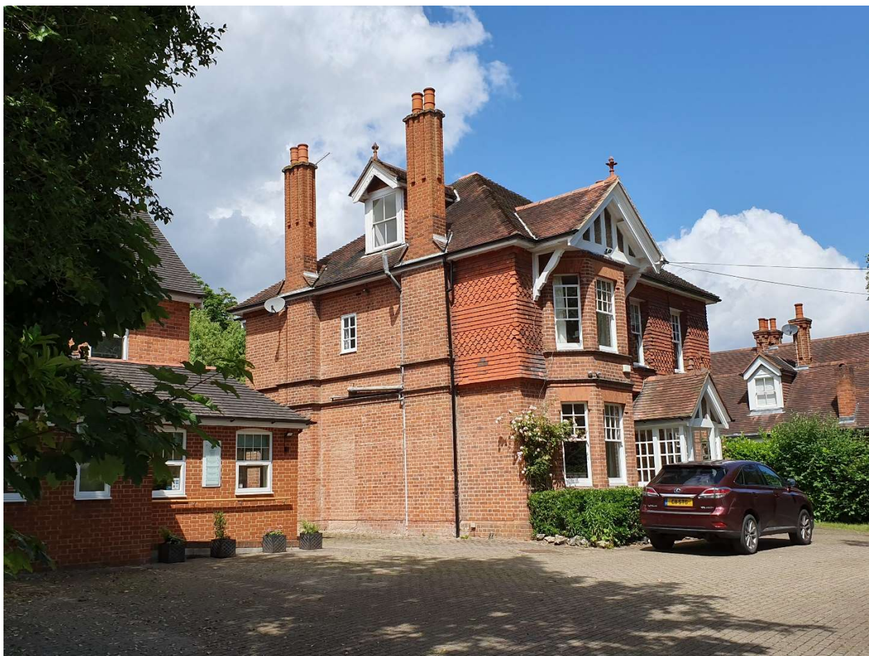
PHOTO No.878-06: 27 & 29 Kidmore Road viewed from SE. High eaves large roof high ridge.
