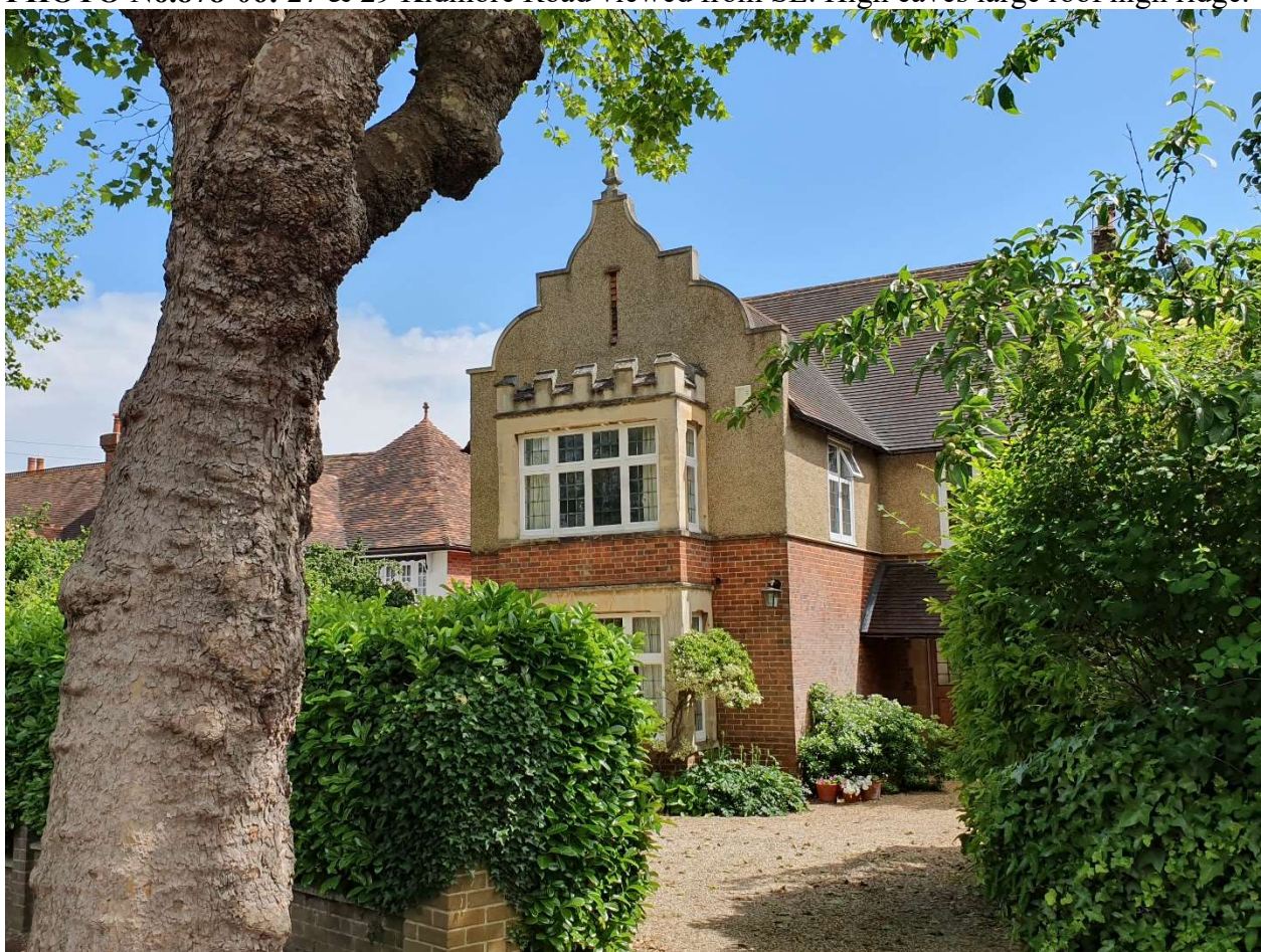
PHOTO No.878-07: 28 Kidmore Road opposite the site. Large roof, high ridge.
