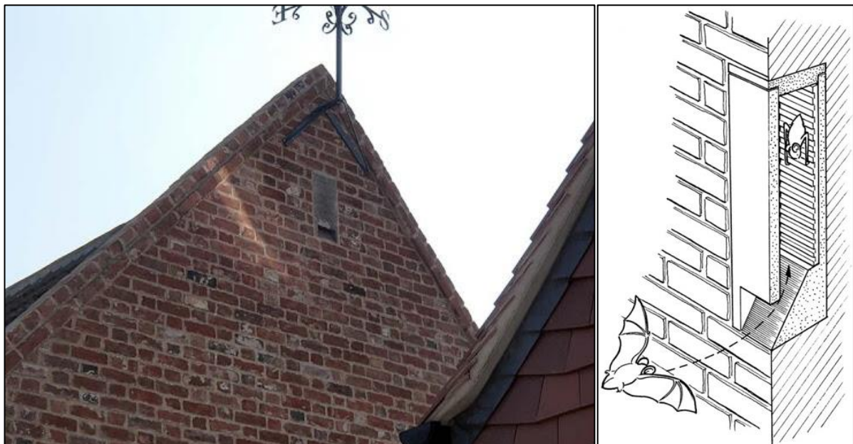
Figure 14. Left – A bat tube integrated into a brick wall. Right – a cross section diagram of a bat tube.
