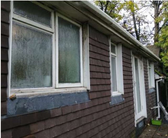
Image 13: Hanging tiles on upper storey of the eastern aspect of the building
