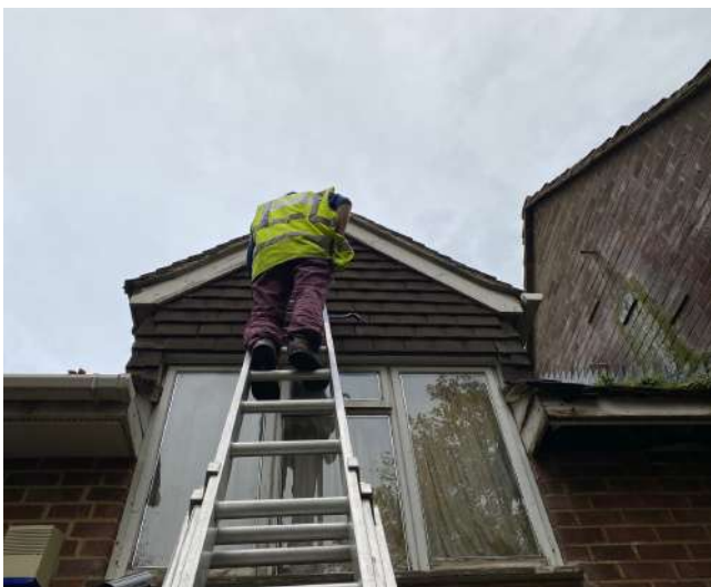
Image 3: Endoscope inspection of hanging tiles at the western elevation
