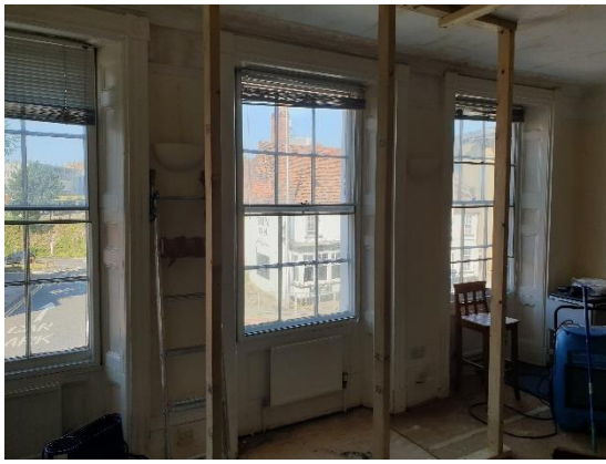
Front classroom wall plaster
