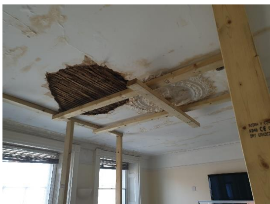
Front Classroom ceiling
