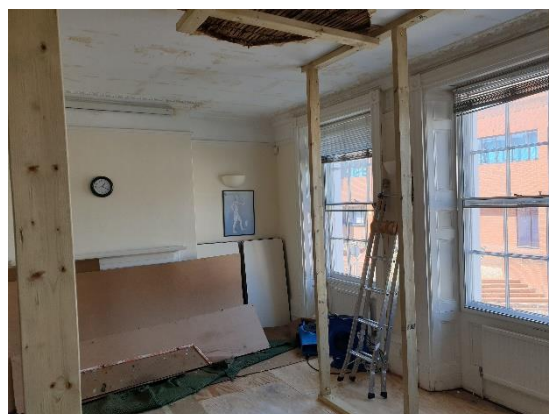
Front Classroom ceiling
