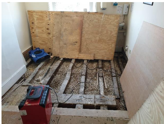
Existing plywood floor lifted to aid drying
