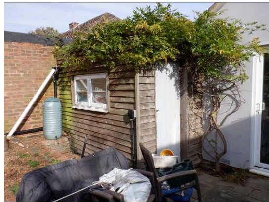
14. Northern side extension (rear/southern elevations).
