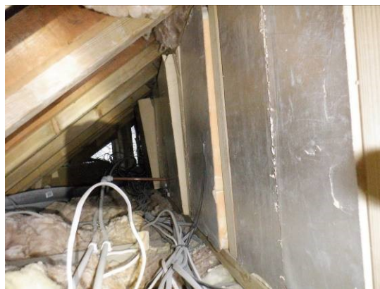
20. Foam insulation boards.
