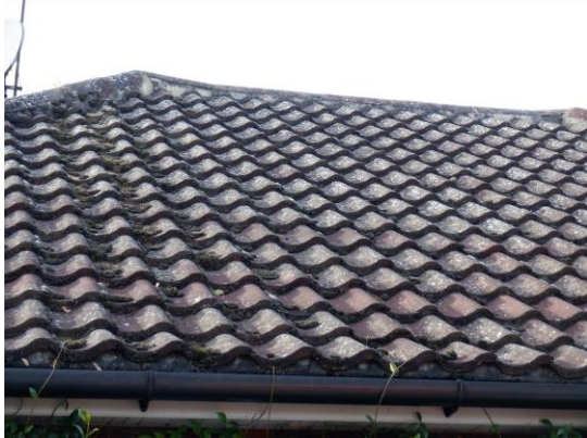
3. Tight interlocking roof tiles (front elevation).
