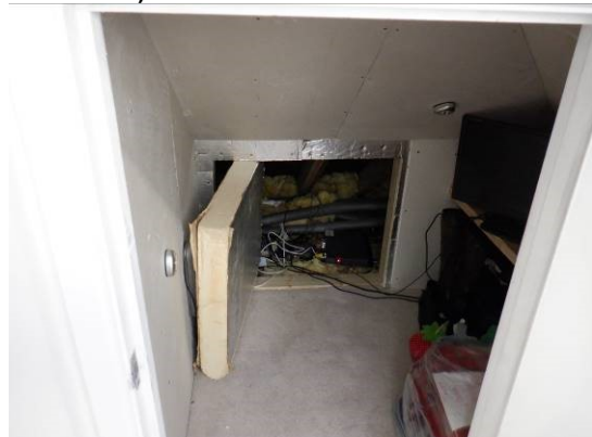
16. Access into eaves space through storage cupboard.
