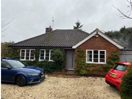
1. Front of property viewed from east.
