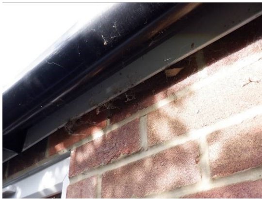
13. Flush uPVC barge board on side extension (southern elevation).
