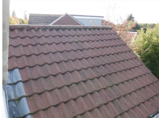
4. Tight interlocking roof tiles on rear extension (northern elevation).
