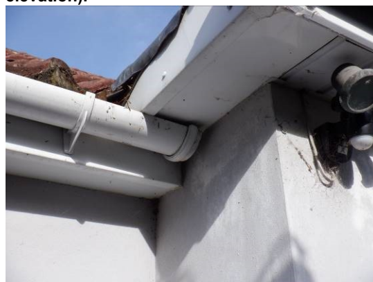
12. Flush uPVC soffit boxes (southern/rear elevations).
