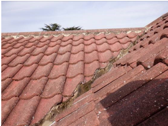
5. Securely mortared ridge tiles on rear gable end (southern elevation).
