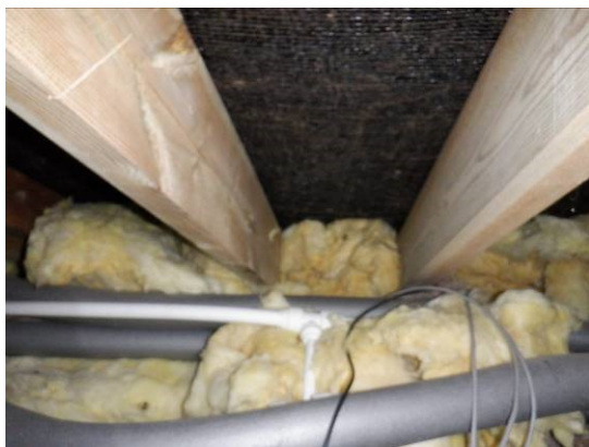
19. Fibreglass insulation leading down into eaves.
