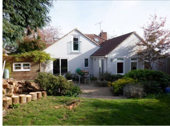
2. Rear of property viewed from west.
