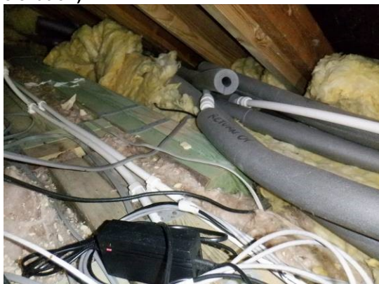
17. Cables and pipework running through eaves space.
