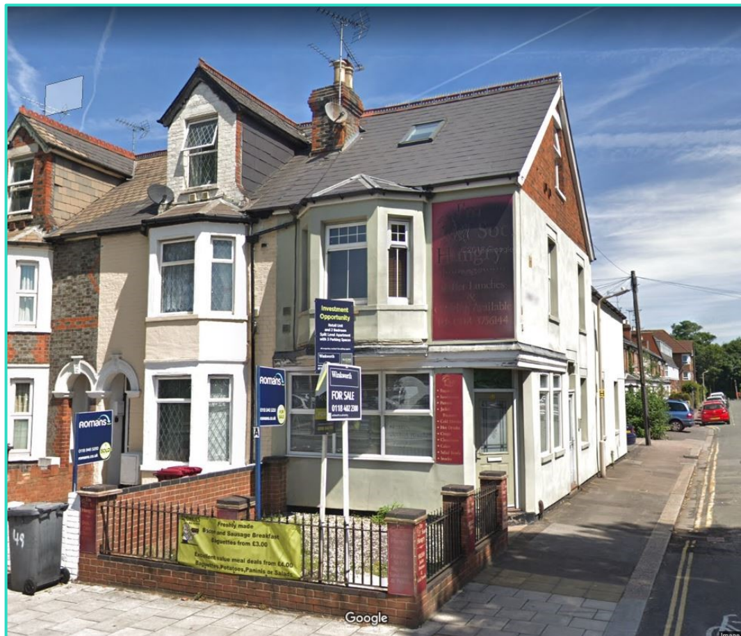
Plate 04 – The Commercial Property at 51 Vastern Road and the Door Light Arrangement above the Front Entrance Door
