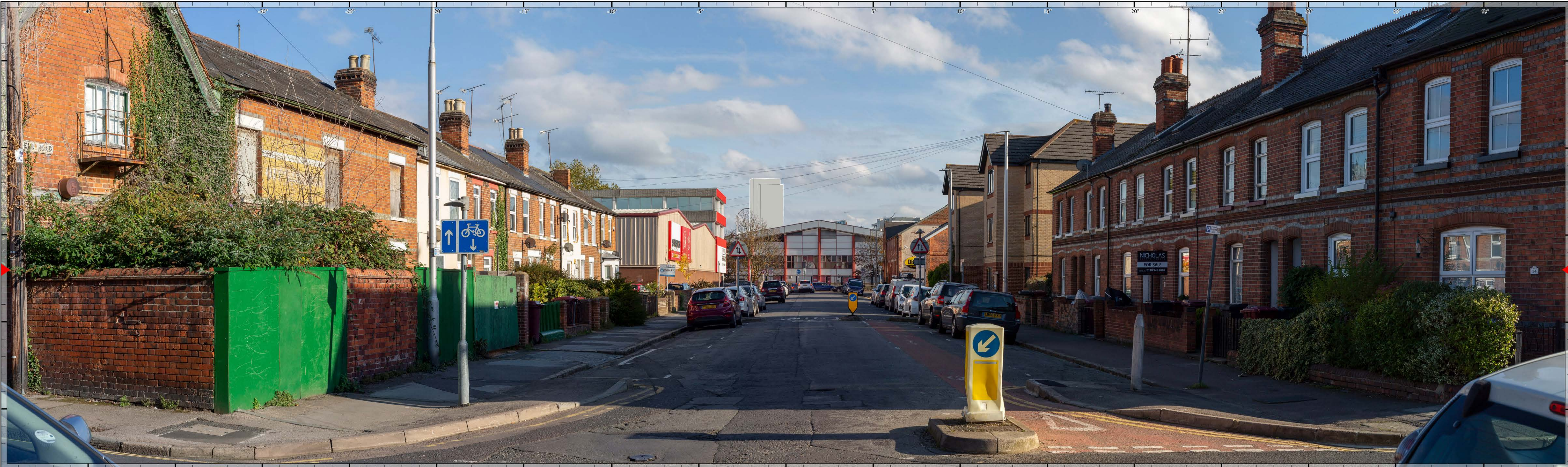
View 17 Swansea Road looking SE - Existing
