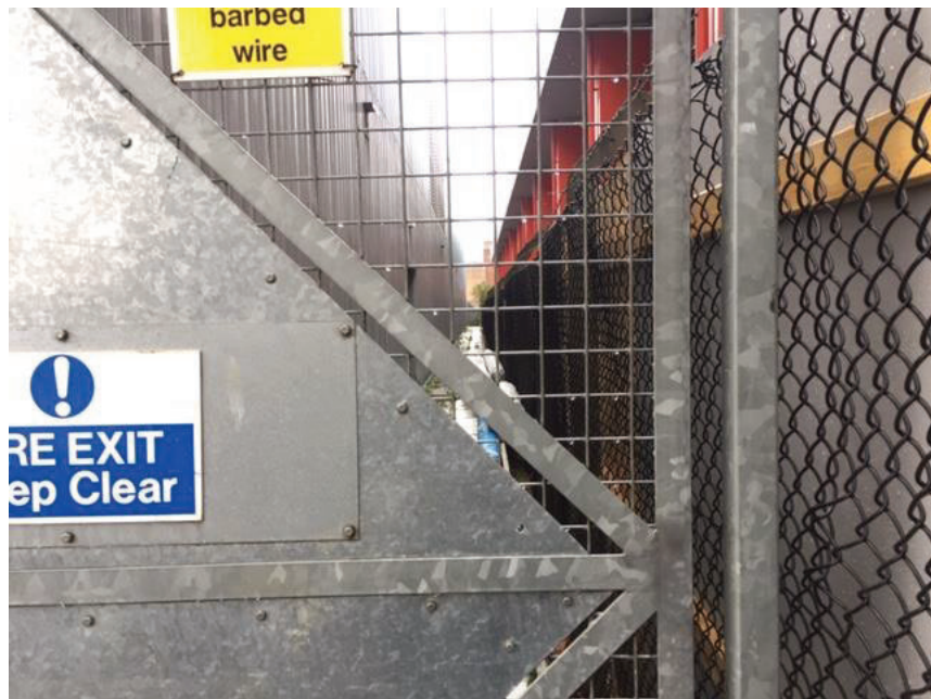
Photo 6. Rear of Building 1, marked as TN1 on Appendix 1, Figure 1
