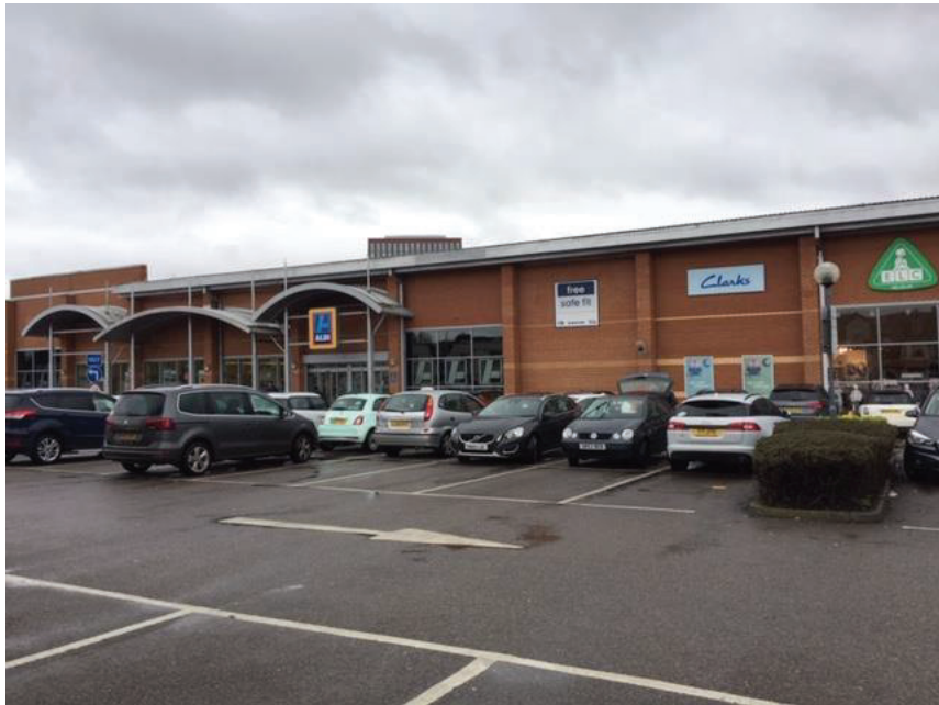
Photo 1. Building 1 (background) and hard standing (foreground)
