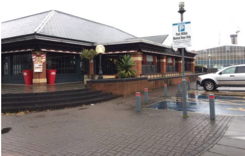
Photo 3. Building 2 (background) and hard standing (foreground)
