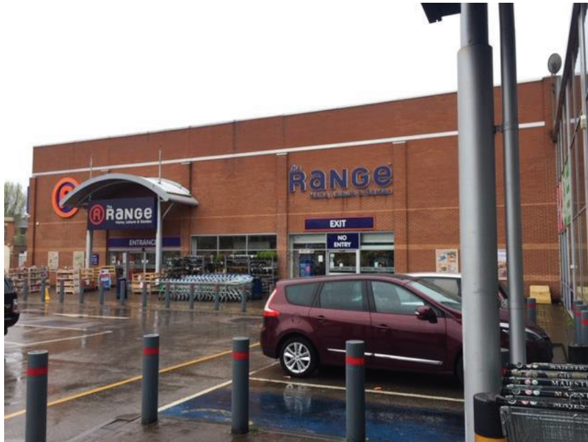
Photo 2. Building 1 (background) and hard standing (foreground)
