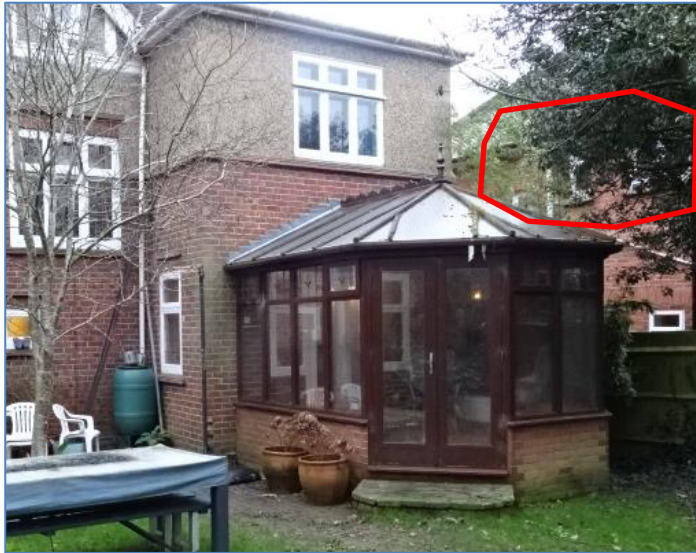
1. Photograph taken on 31/01/2020, supplied by agent. Red outline demonstrates side elevation windows at 59 Peppard Road
