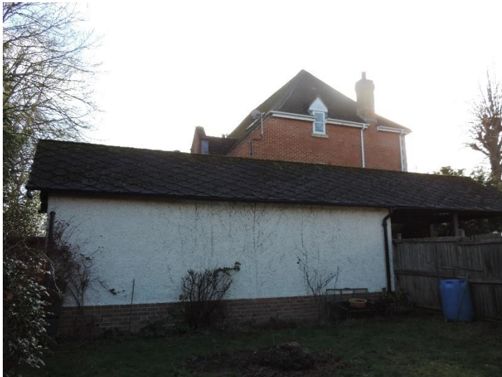
Plate 8. Typical view of the garage.
