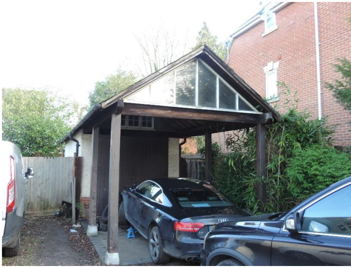
Plate 7. Typical view of the garage.
