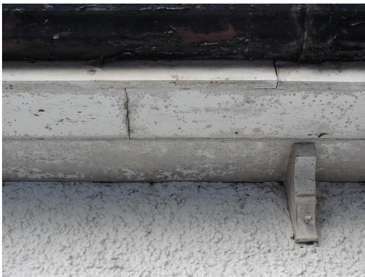
Plate 6. Typical view of the soffit and fascia.
