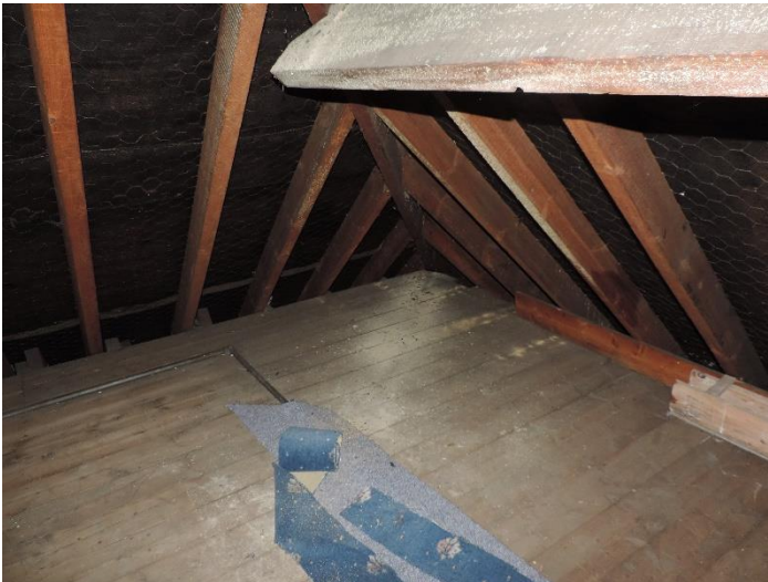
Plate 11. Typical view of the eave void space.
