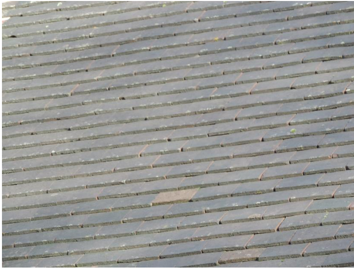
Plate 4. Typical view of roof tiles.
