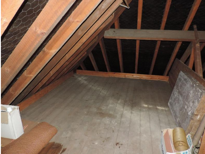
Plate 10. Typical view of the eave void space.
