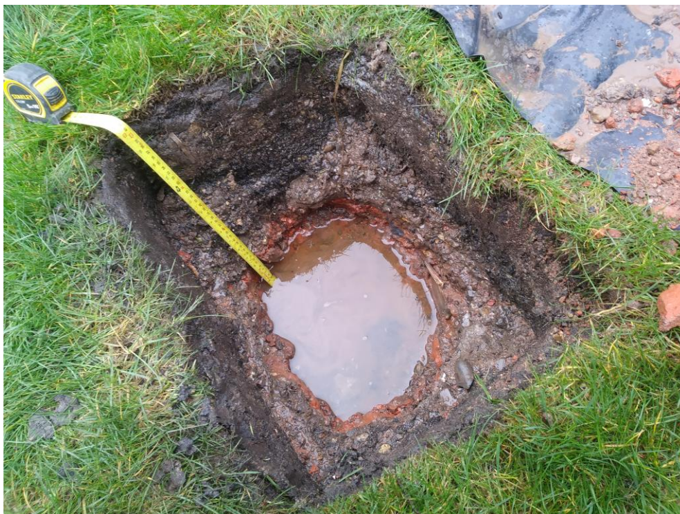
Photo 22: TP103 – membrane at 0.42m
