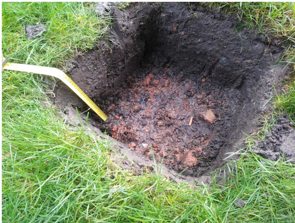
Photo 16: TP102 – membrane at 0.36m
