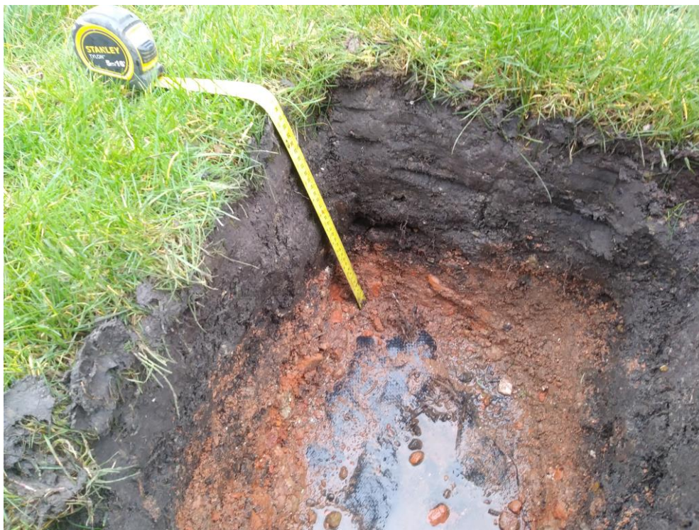
Photo 18: TP102 – membrane at 0.36m
