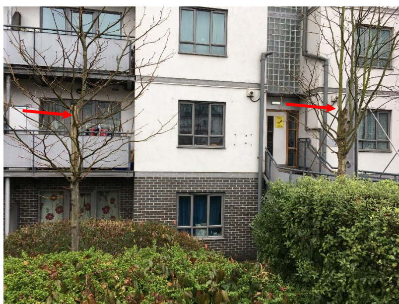
Photo 2 – Trees T6 & T7, arrows indicating point of damage and loss of original leaders
