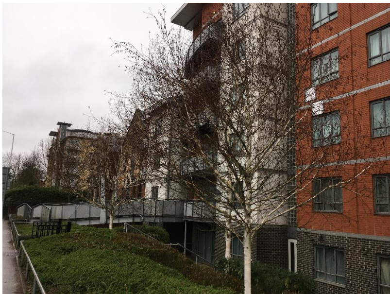
Photo 1 – T1 & T2 are located the far side of the footbridge, with T3-T5 in the foreground
