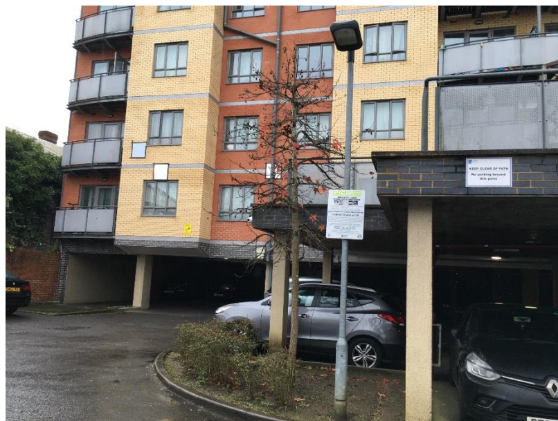
Photo 5 – T17 looking south, towards the rear of the building
