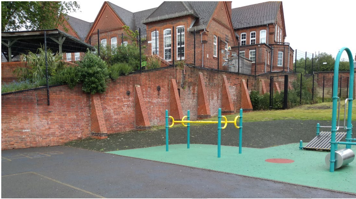
Fig 5: South facing elevation of retaining wall showing modern buttresses.
