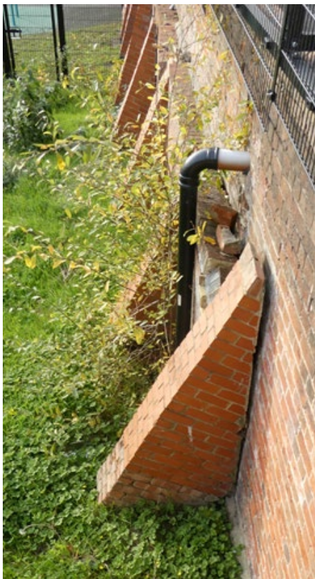
Fig 6 & 7 : Detail of detached moderns buttresses to south facing retaining wall.
