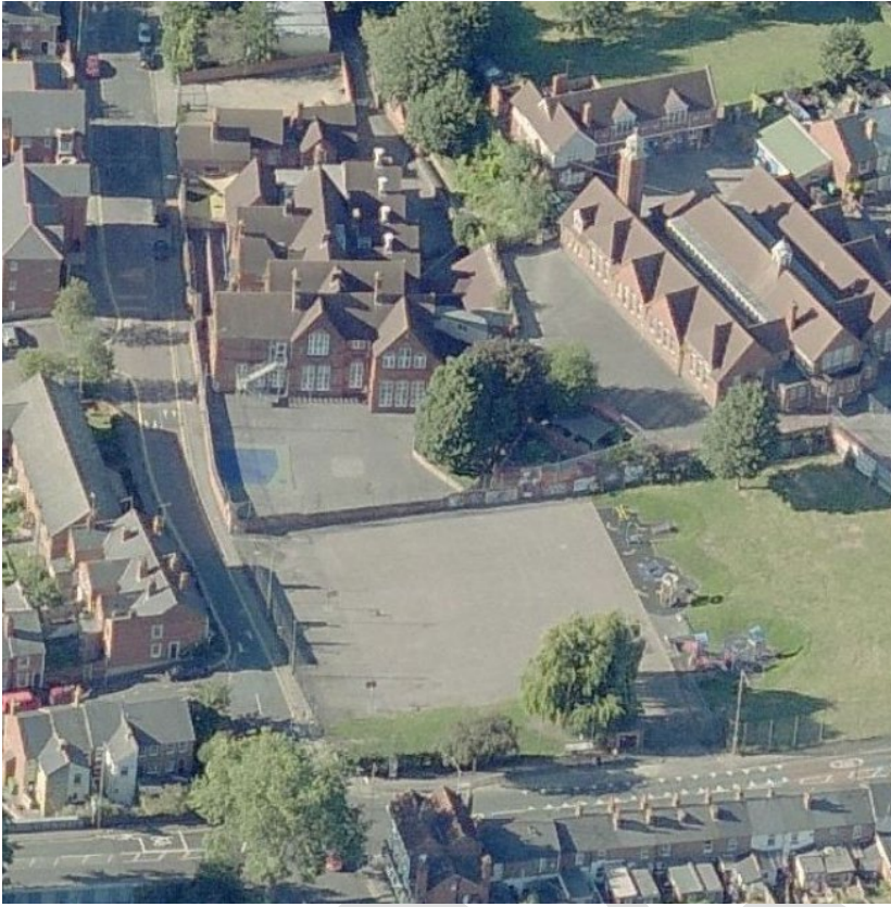
Fig 1: Aerial view of South elevation of Henry Building with retaining wall in the foreground
