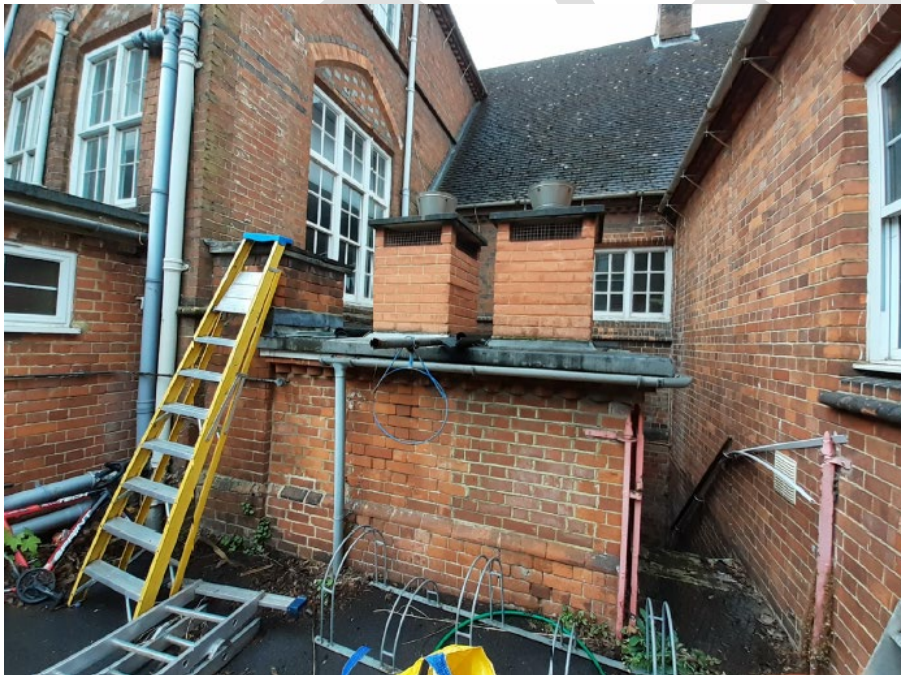
Fig 10 : Existing plant room area (East facing)
