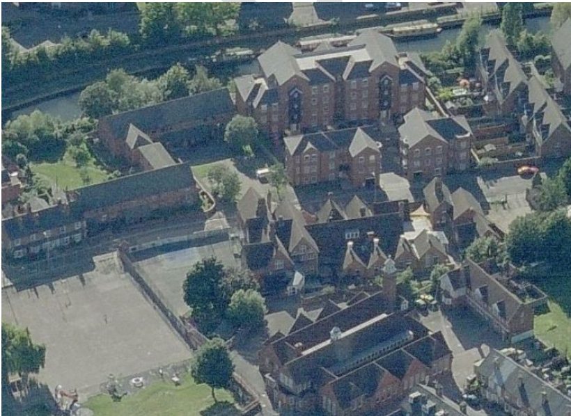
Fig 2: Aerial view of West elevation of Henry Building
