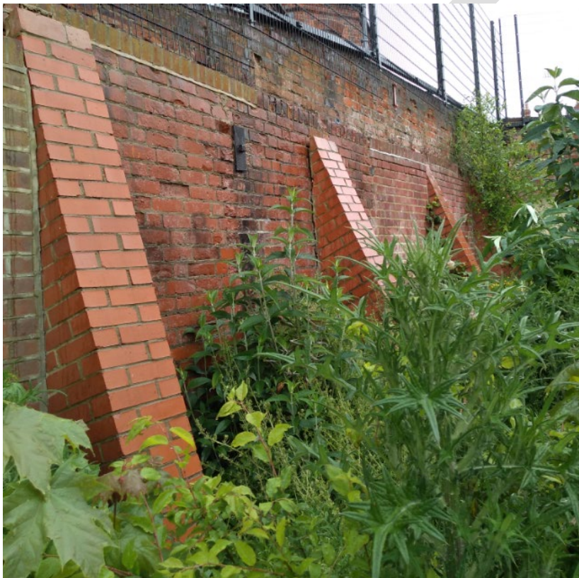
Fig 9: East end of south facing wall, showing modern single leaf facing brick to right hand side.
