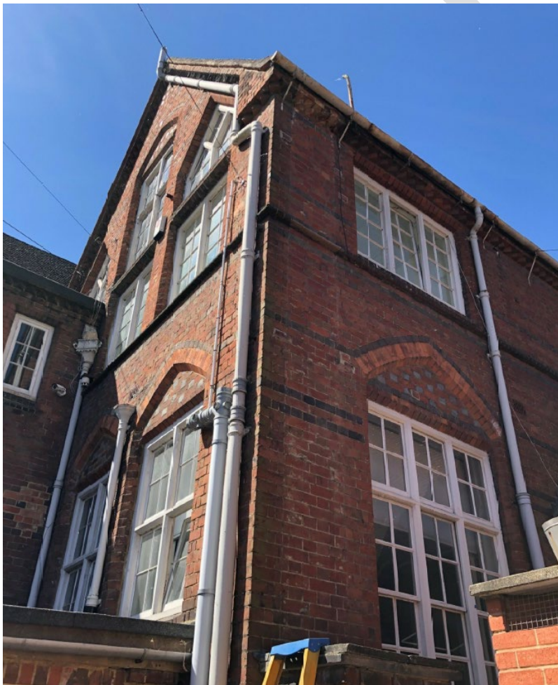
Fig 4: East Facing Gable, line of former flue visible on north facing return brickwork
