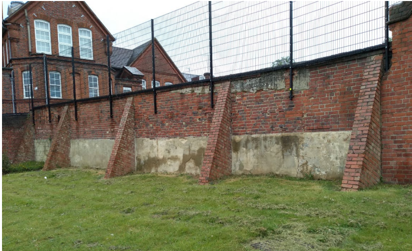
Fig 8: West facing return wall.
