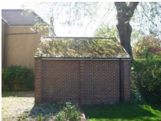
47. Garage roof (northern elevation).
