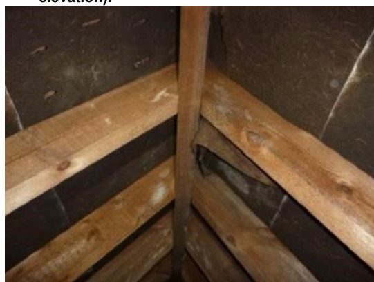
56. Internal roof space felt roof with timber beams.
