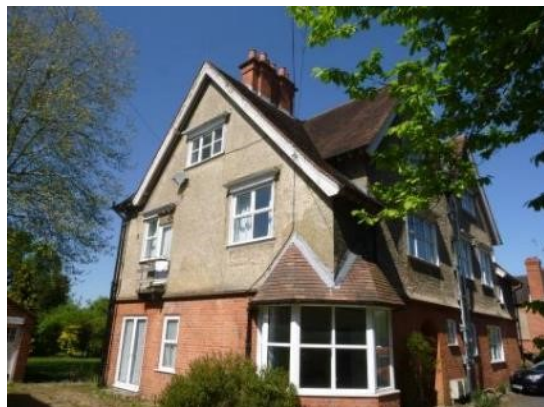
2. South-eastern elevation of the house.
