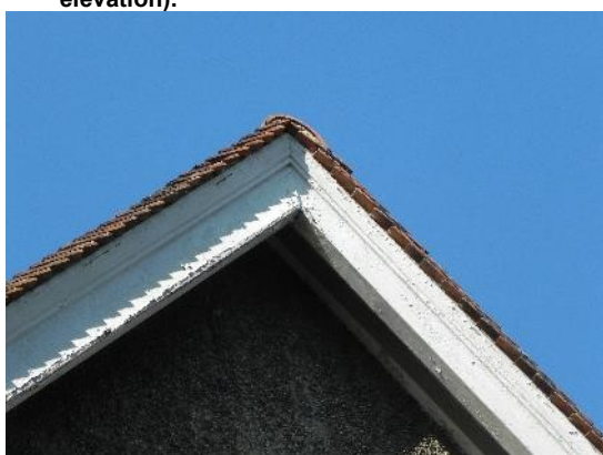
29. Gap to gable apex (northern elevation).
