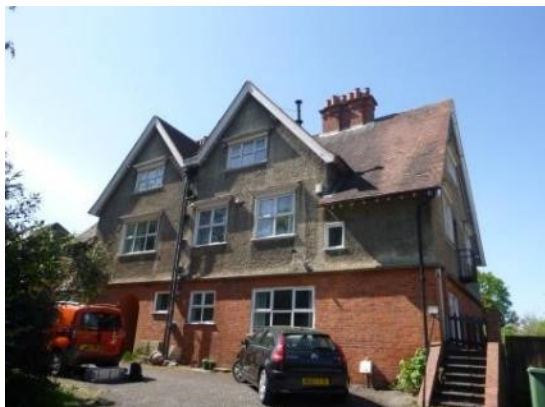
1. North-eastern elevation of the house.
