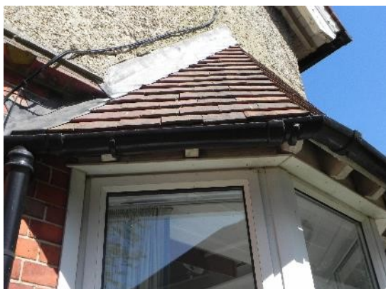
39. Tiles lifted to edge of bay window roof.
