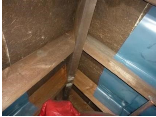
58. Internal roof space - sheeting covering gaps in felt.
