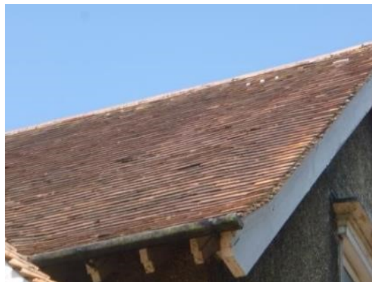
34. Tiles lifted to gable (south-eastern elevation).
