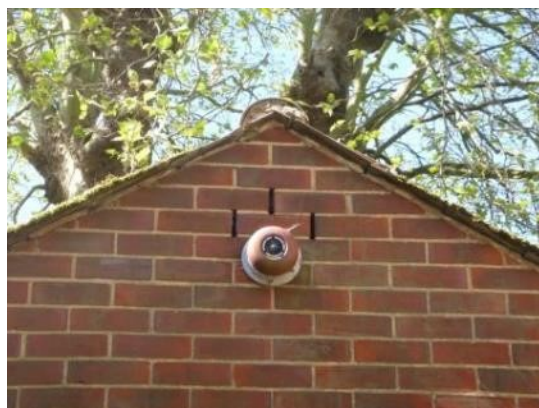
46. Weep holes between bricks in garage.
