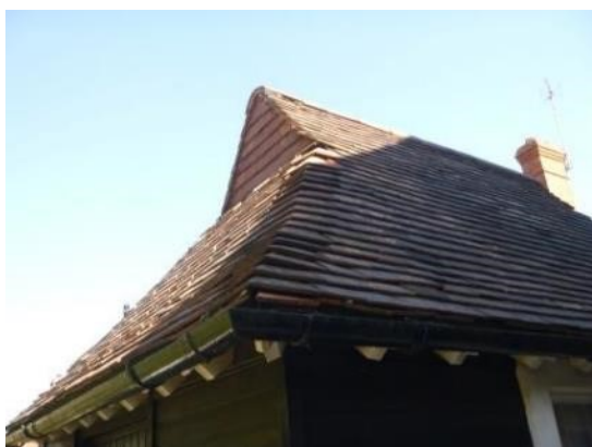
51. Shed tiles lifted down hip (south-eastern elevation).
