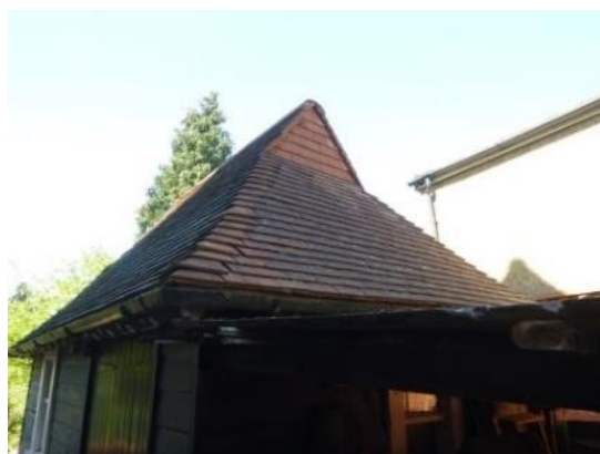
52. Shed tiles lifted down hip (south-western elevation).
