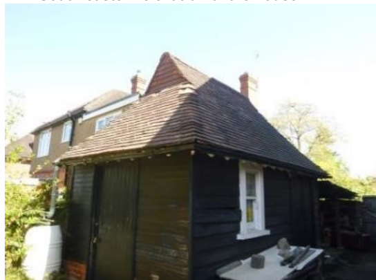
4. South-western elevation of the shed.
