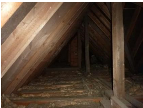
55. Internal roof space cut-and-pitch construction with fibreglass and boarded flooring.
